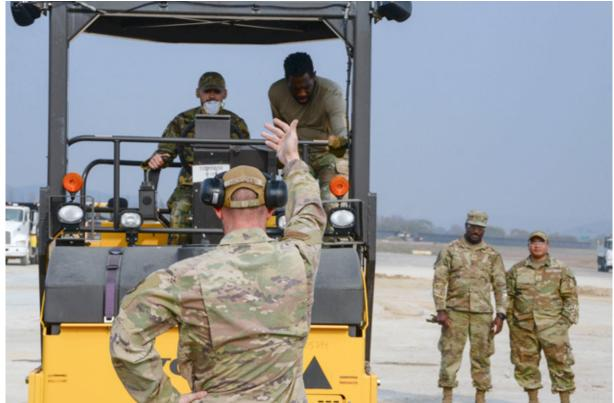
U.S. Air Force Airmen assigned to the 51st Civil Engineer Squadron, roll and flatten freshly poured asphalt to repair a simulated crater at Osan Air Base, Republic of Korea, April 3, 2025. The efforts were part of a daylong instructional and hands-on rapid airfield damage repair training to educate and prepare participants for the upcoming joint and combined IRON RADR exercise hosted by the 51st CES.
